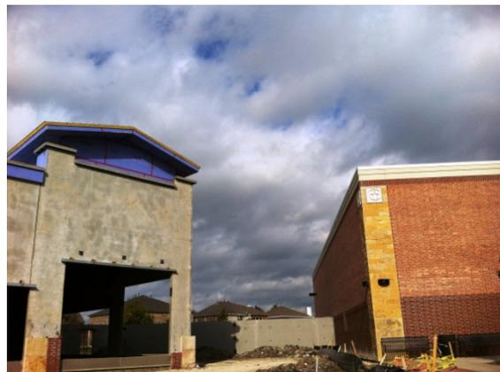
Tilt wall before and after being covered with true masonry materials laid up unit by unit by a mason and set in mortar. The Kroger shopping center in McKinney, Texas.
