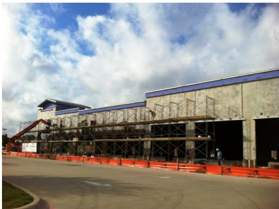
Tilt wall construction being covered by true masonry. The Kroger shopping center at El Dorado and Custer Road in McKinney, Texas
