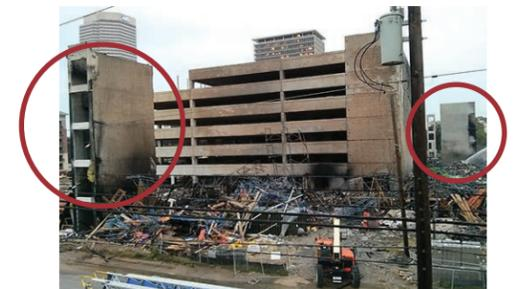
In the Axis apartment fire in Houston, as in most multi-unit residential fires, the only walls left standing were the masonry walls – stair wells and the adjacent parking garage.
